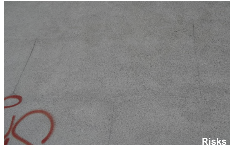
Shrinking of the plaster
