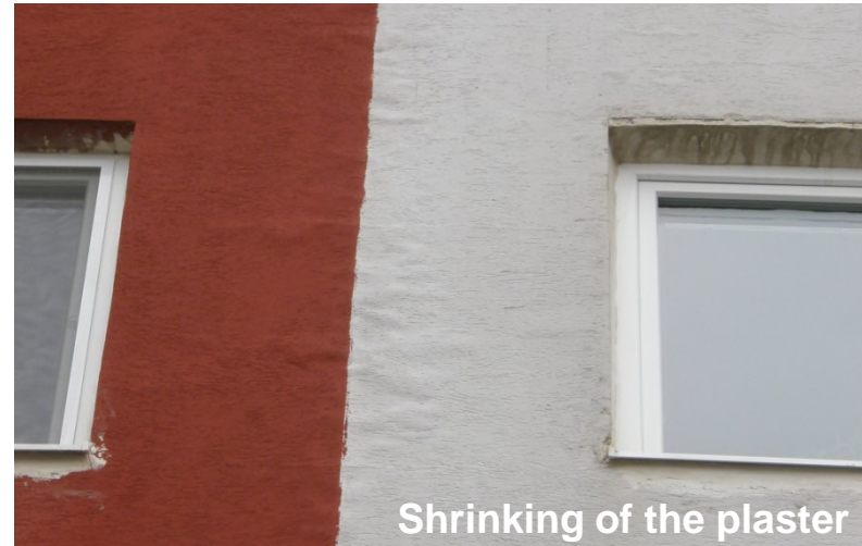
Shrinking and separation of plaster
